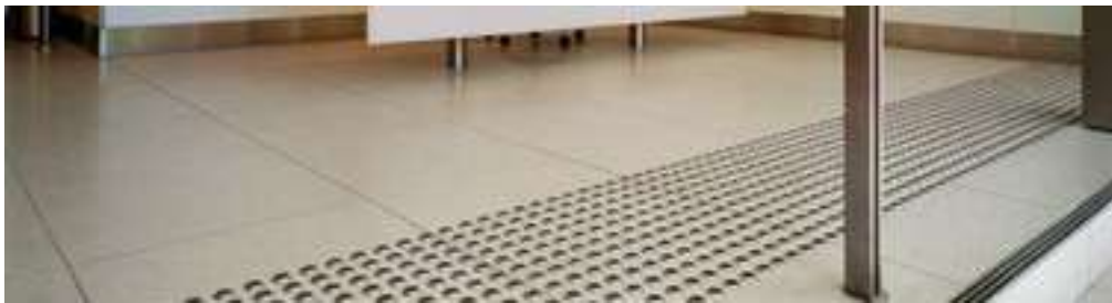
DTAC DT0200 INSTALLATION
