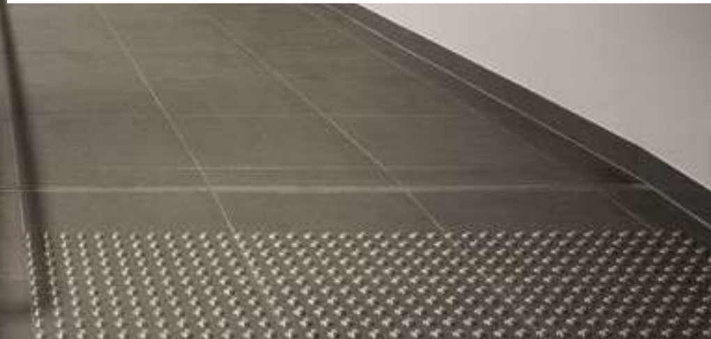
DTAC DIT0010 CLASSIC INSTALLATION (INTEGRATED)
