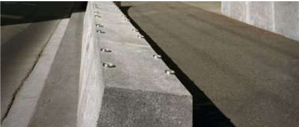
DTAC DEP0010 INSTALLATION
