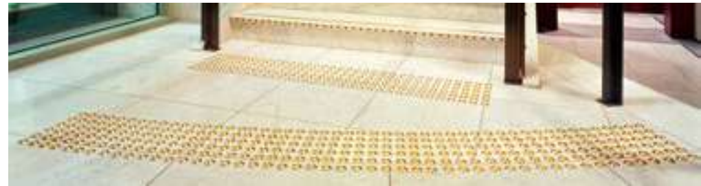
DTAC DT0300 INSTALLATION
