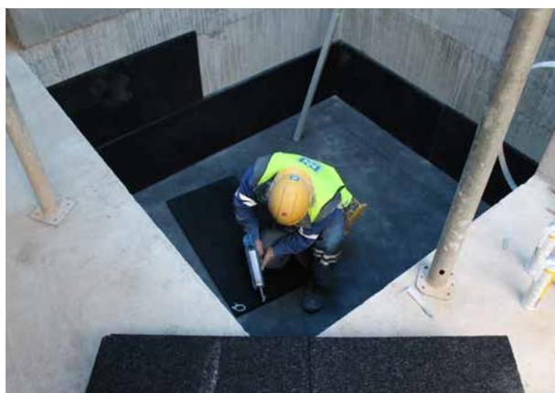
two technical engineers were sent to the site by BSW to supervise the installation work on site and ensure assistance. After completion of the installation, the vibration control **Regupol®** insulation layer was then built over by the overlying storeys during the course of the construction activity and thus became a technically effective component part of the building foundation.
